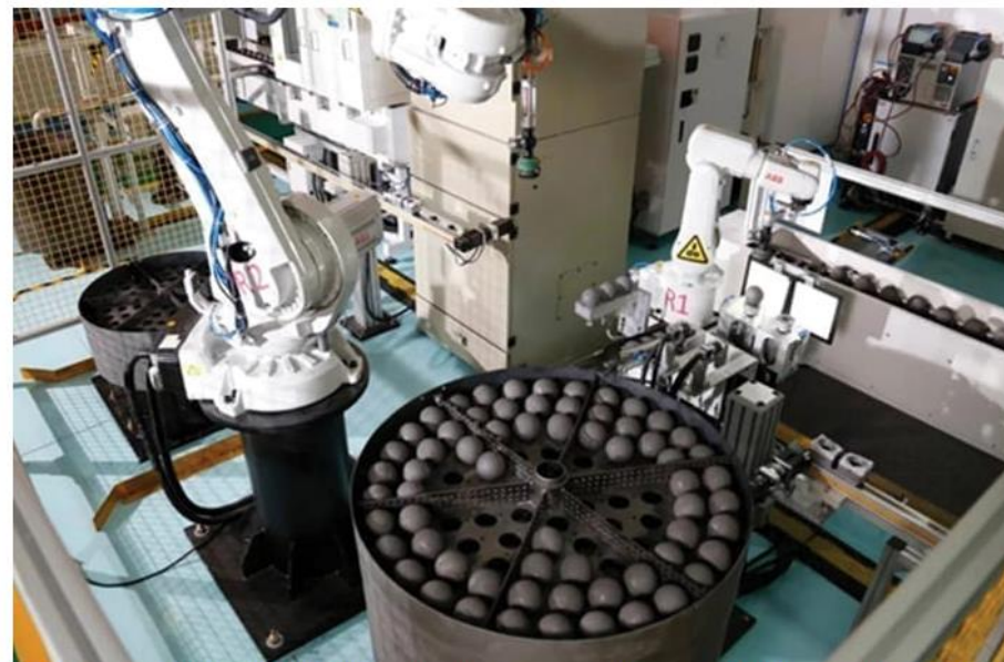
Fuel loading at the Shidaowan high-temperature gas-cooled reactor pebble-bed module (HTR-PM) in China began in the spring of 2021. It involved putting 870,000 spherical TRISO fuel elements into the two small reactors that will drive a single 210-MWe turbine. Courtesy: China National Nuclear Corp. (CNNC)
