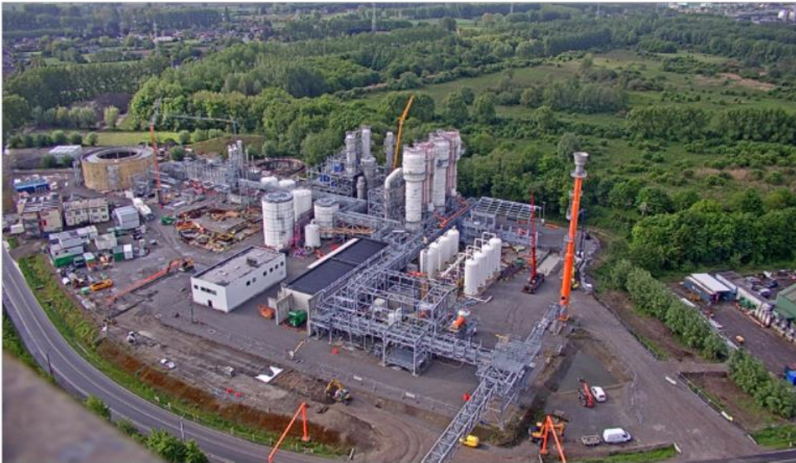
Fig. 25: Construction of the Steelanol plant at ArcelorMittal Gent 26
